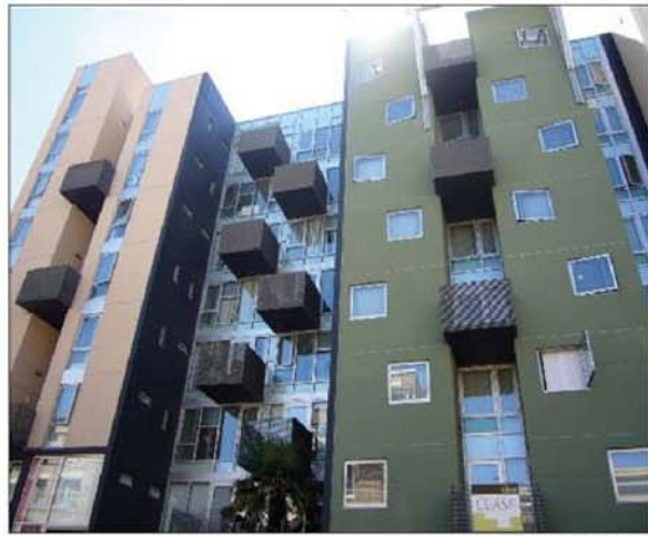
The Curran House, at 145 Taylor St., has earned a local architecture firm an award.
