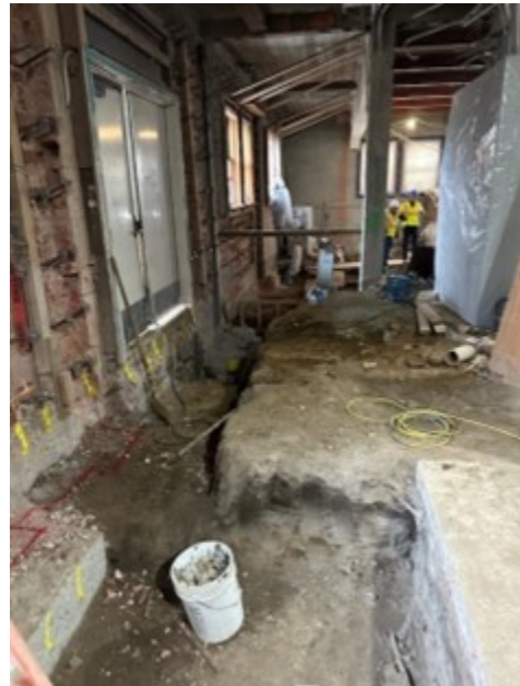
Community room, interior demolition.
