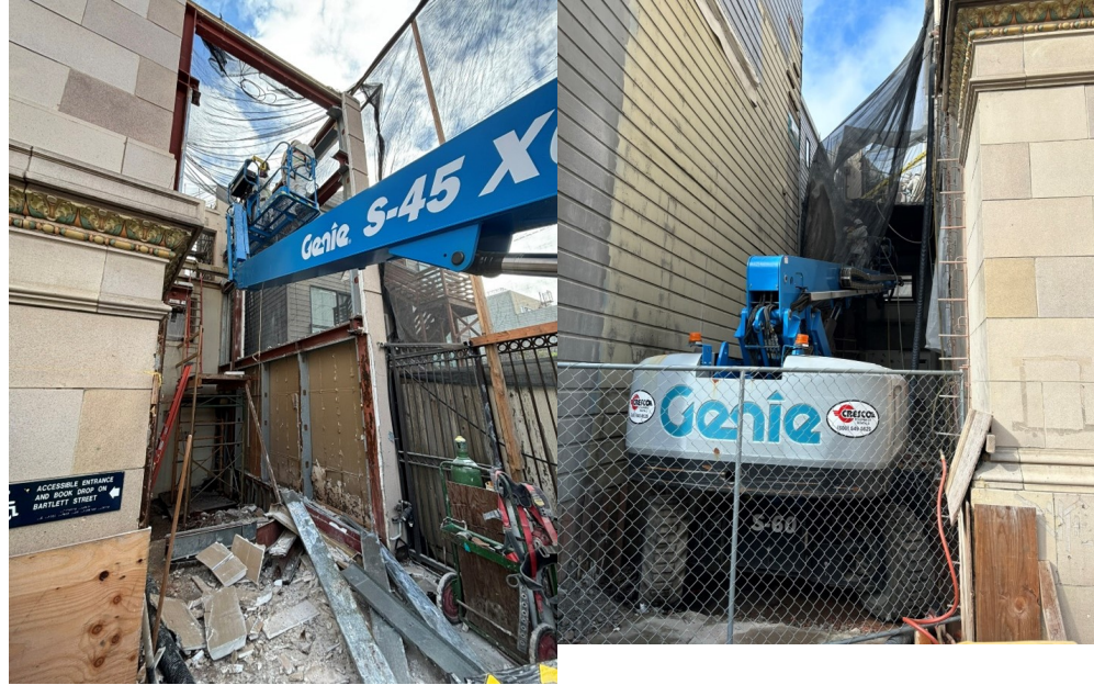
View from Bartlett Street - south wall demolition.
