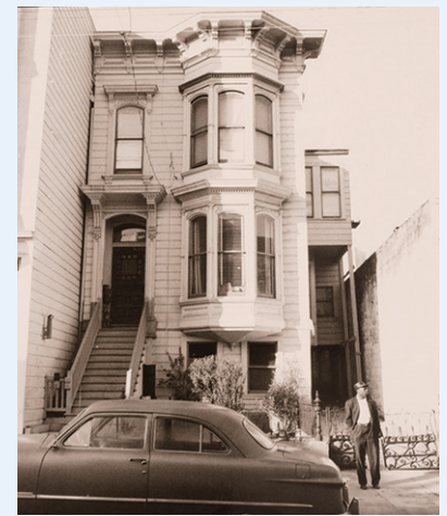
1804 Ellis St., 1962. Appraisal Report of San Francisco Redevelopment, Area A-2, Western Addition, Vol 5. SFRA Records, San Francisco History Center.
