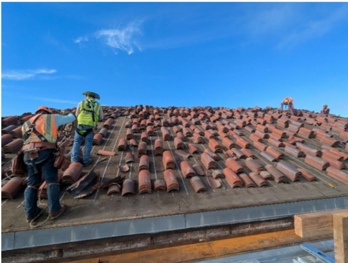
View of the north-facing side showing tile roof repair and replacement.
