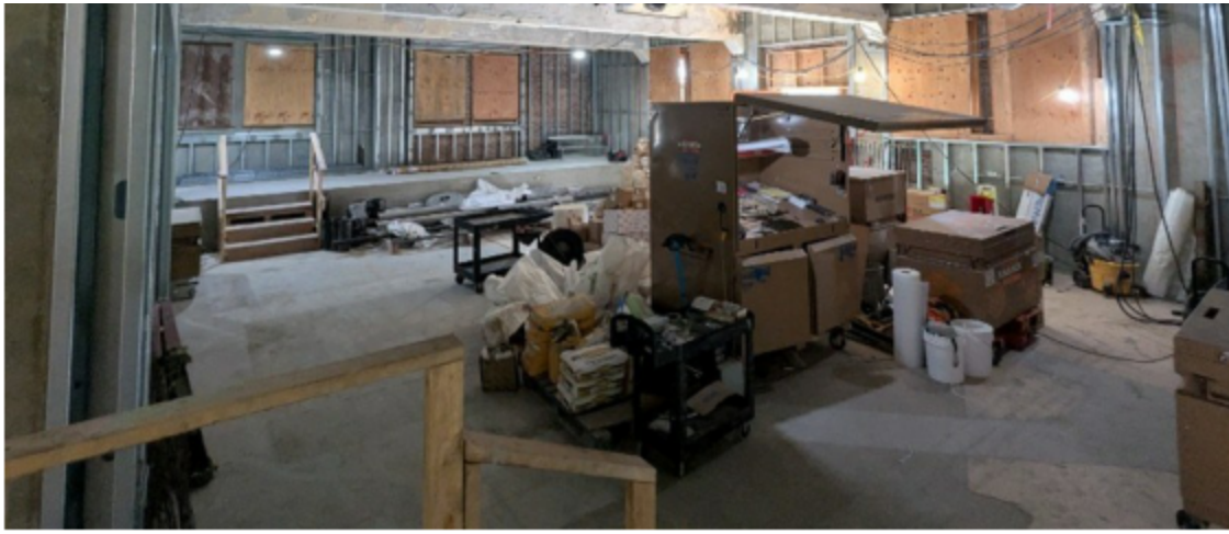
Interior view of the new Community Room.
