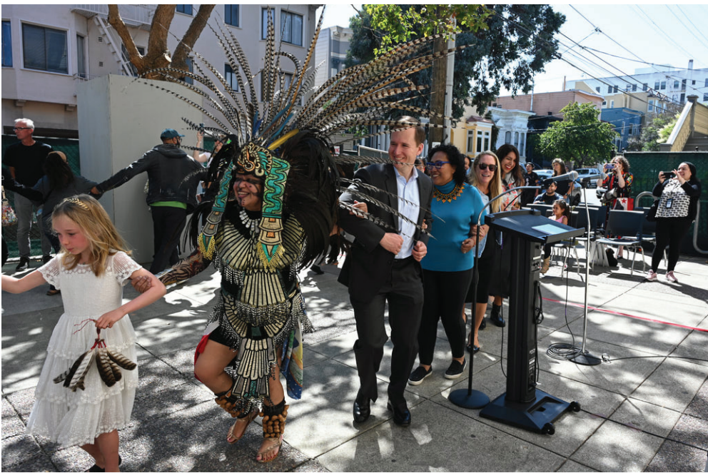
Photos: Top: Library staff, Library Commissioners, Friends of the Library staff, Friends Board members, City architects and community partners on a hard-hat tour of the Mission Branch renovation site. Bottom: Celebration at the groundbreaking ceremony in 2023.
