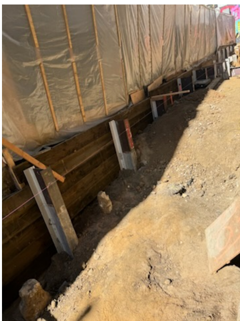
Exterior view from Bartlett St. — Adjacent building, underpinning
